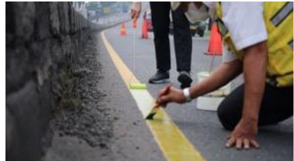
Gambar 6. Pengaplikasian lapisan marka glow in the dark
