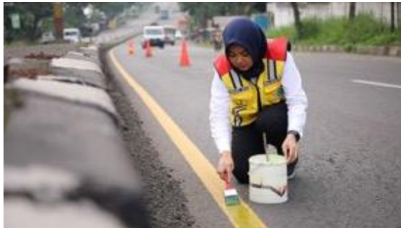
Gambar 6. Pengaplikasian lapisan marka glow in the dark
