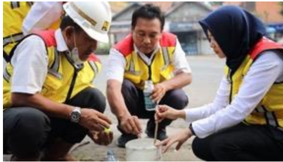
Gambar 5. Proses pencampuran larutan marka glow in the dark
