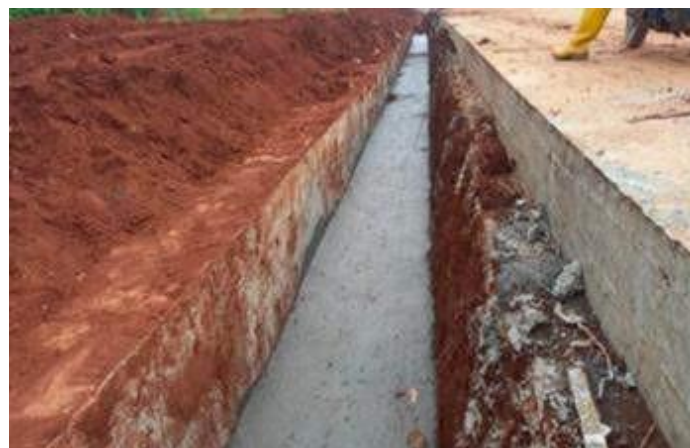
Gambar 6. Pengecoran lean concrete
